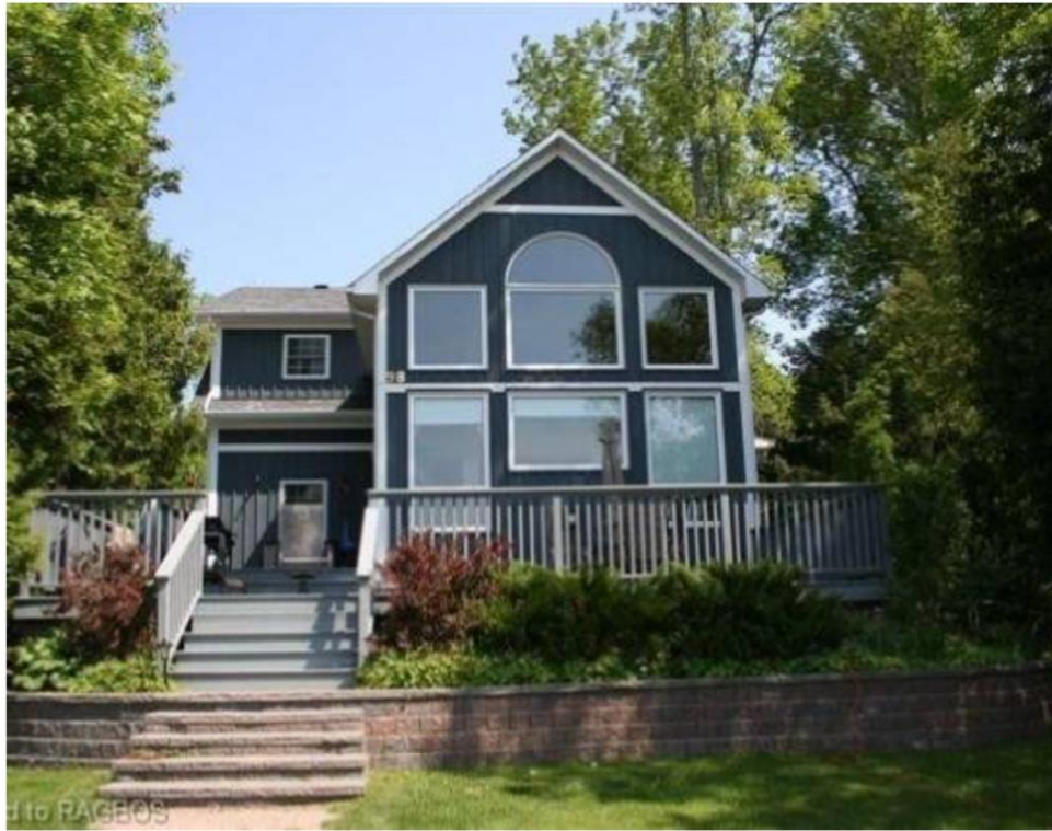
98 Bruce Beach Road – Front Yard (Lake Side) 2014 (above)
